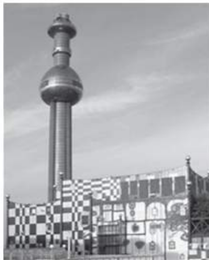
Figure: Incineration plant
